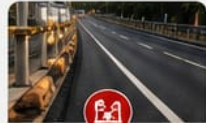
ROAD CONSTRUCTION & MAINTENANCE
